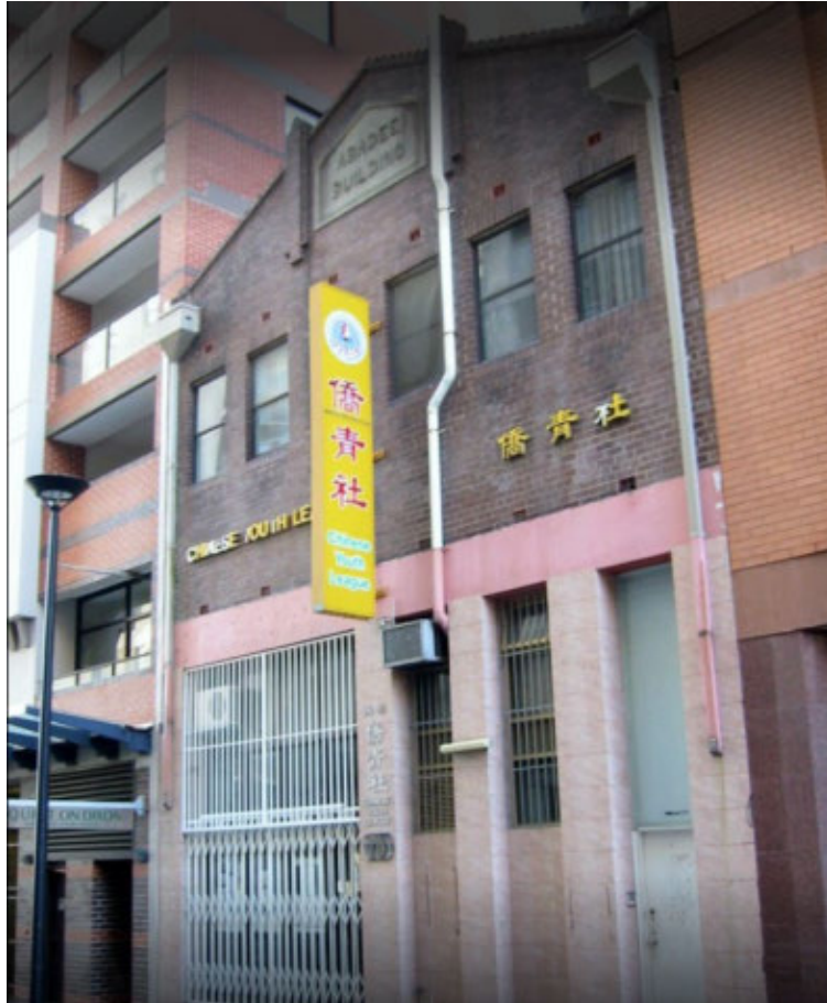
10 Dixon Street. The building was donated by the Wran Government to the Chinese Youth League for use as their clubhouse. (Source: The China–Australia Heritage Corridor)
